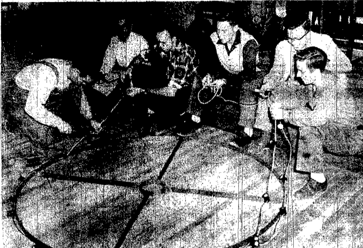
Members of the Wayne Jaycees are pictured above working on new Christmas street lighting decorations which will go on in Wayne Nov. 24. Jaycees were busy this week getting the 50 units ready for installation on light poles throughout the business district. Pictured, left to right, are Earl Larson, Alvin Voorhies, Dave Hamer, Chuck Surber, Warren Ruskell and Norman Ellis.
